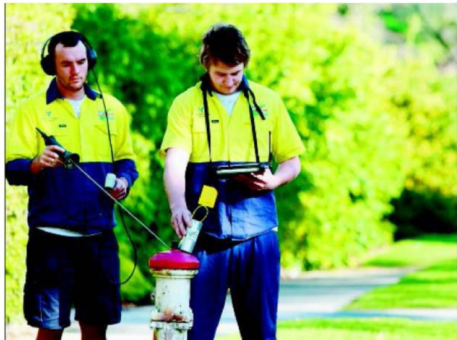
Yarra Valley Water leakage technicians Matt Roff and Mitch Wright at work in Banyule.
